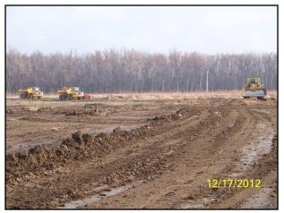
On left, Contractor is placing levee embankment to full height on downstream end of Upper Crevasse. On right, Contractor is building haul road from sand deposited from scour to begin hauling and building landside berm at Center Crevasse.
